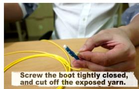
**Screw the boot tightly closed, and cut off the exposed yarn.**
