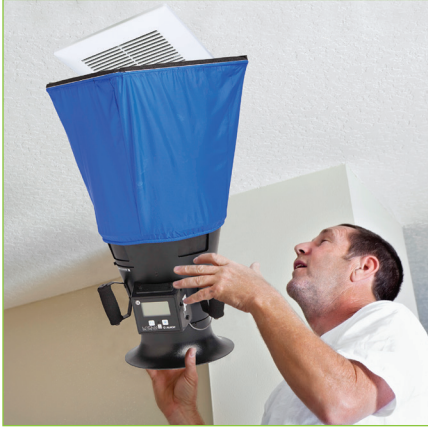
Balometer used to verify installed performance
