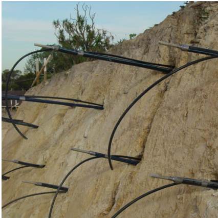
Soil Nails/Anchors prior to grouting.
