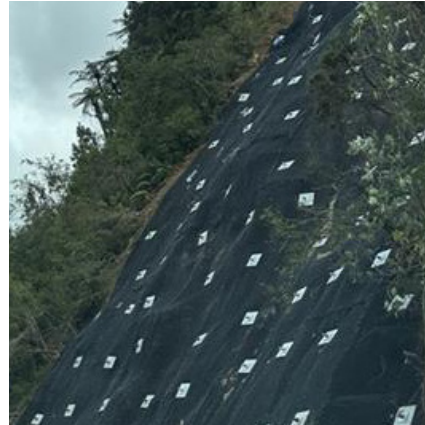
Soil Nails/Anchors post-grouting.
