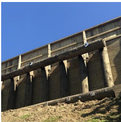
Retaining wall tie back.
