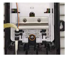
2. Tighten the three screws in the enclosure.
