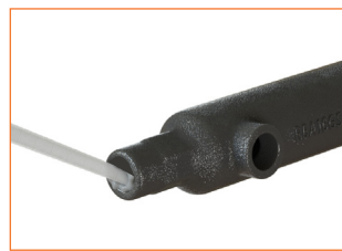
2.c: Dispense remaining half of recommended Epoxy (refer to table above) into threaded end of Grout Sleeve. Ensure even distribution through internal threads.
