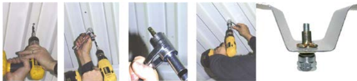
Step 1 Step 2 Step 3 Step 4 Completed Installation
