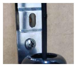
2. If using the drywall anchors, install them 9 in apart. Install the wood screws into the holes onto the lower hole of the mounting bracket.
