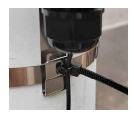
3. Use a large zip tie to attach the cable to the hook of the mounting bracket as a strain relief. Don't forget to cut off the excess zip tie.
