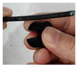
Install the smallest grommet that fits over the outer jacket over the cable.
