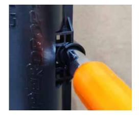
1. Unscrew the embedded screw with a 3/8-inch nutdriver.
