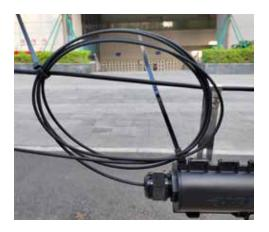
Secure the excess cable to the aerial and the top corners of the enclosure with the large zip ties.
