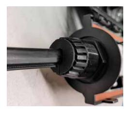
Follow the instructions for the round fiber optic cable using the flat-drop grommet. Verify the flat-drop cable is on the same plane as the splice tray before tightening the sealling nut and the trace wire is outside the grommet.
