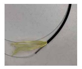
3. Remove 0.5 to 1 m (~1.5 to 3 ft) of outer jacket material and trim the aramid fiber to 30mm (~1 1/4 in).
