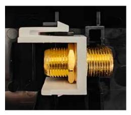
The squeezable tab on keystone jacks must be fitted between offset supports to keep the patches aligned.
