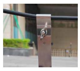
2. After hanging the enclosure from the aerial, use the screws with blue threadlocker and wingnuts to secure the enclosure.
