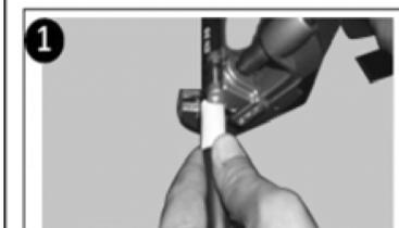
**1:** Measure the suitable length of cable before peeling (ensure the cable can reach the furthest splice tray), mark on the cable jacket with knife (make sure not to damage the fiber).
