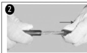
**2:** Remove materials surrounding the cable strip and the bundle tube, expose to fiber optic, clean the reinforcement core, keep suitable length for fixture.
