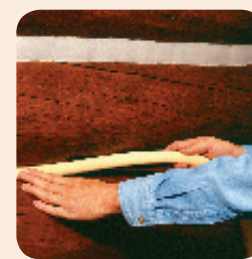
2. Or, install backer rod into caulk well of clean, stained logs.
