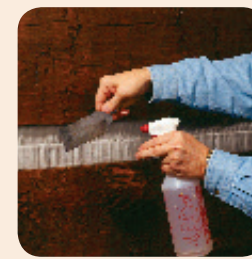
4. Lightly mist the trowel as needed.
