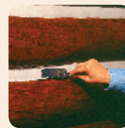
5. Tool to ensure a tight seal to the top and bottom of the chink line.
