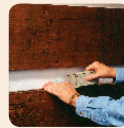
2. Tape the entire joint using polyester tape.
