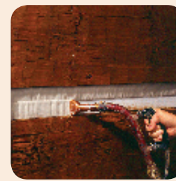
3. Gun Log Jam® over the backer material.
