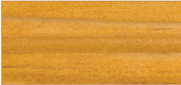
Wood was stained, then caulked.
