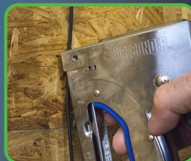
Secure 1meter of cable with 20 staples on a wood panel
