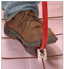
Protective plastic-to-plastic PEX connections.
