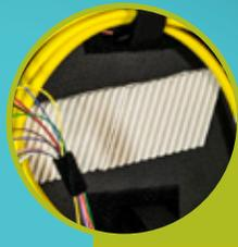
**Grommeted Non-captive Entry Portals** - Protects cables from sharp edges and makes future moves, adds and changes easier
