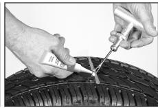
of the plugger needle. Coat the middle section of the tire plug with Plug Bond.
