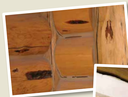
Cohesive failure of chinking
