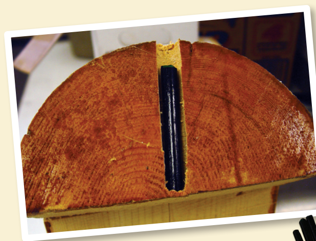
Log cross-section showing an installed borate rod.
