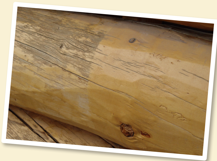
1 coat (left) vs. 2 coats (right) – it makes a difference!
