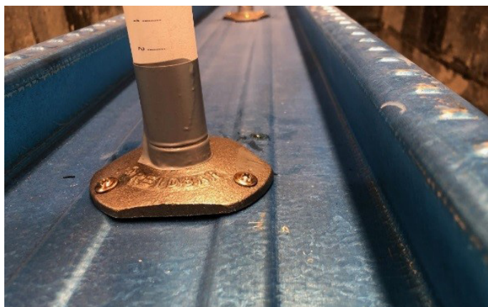
Figure 3 – Testing installation of Rapidbrace system onto steel profiled decking.
