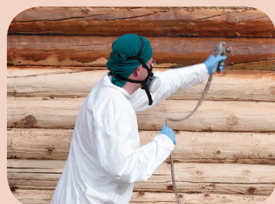
Spray on stain using a *Graco® 515 or 313 tip or equivalent.
