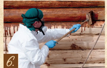
Apply Wood Preservative
