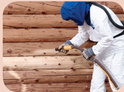
Corn Cob or Glass Blasting (Recommended method)
