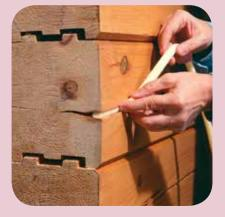
1 – Install backer rod into a clean, stained check to the appropriate depth. (See Fundamental Application Guidelines.)
